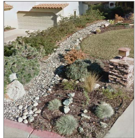
Install rain gardens and dry swales, and augment soils, to enhance infiltration, disperse flows, and detain runoff at low-permeability sites.
