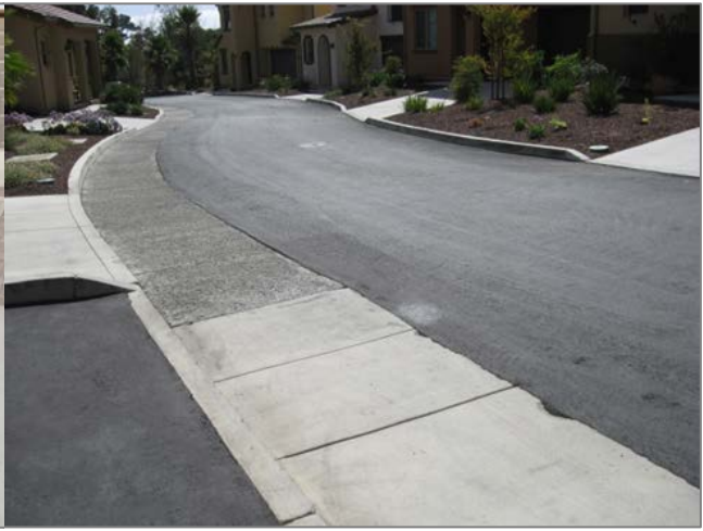
Using permeable concrete for gutters, sharing driveways, and minimizing street dimensions all decrease the impervious surface area in housing developments.
