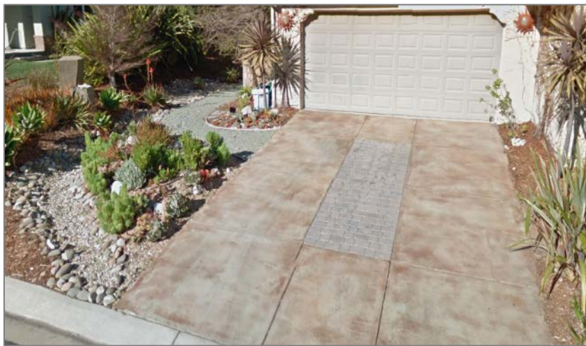
Decomposed granite, permeable pavements, and dry swales compliment the drought-resistant landscaping (with minimal chemical maintenance required) at this SFR.
