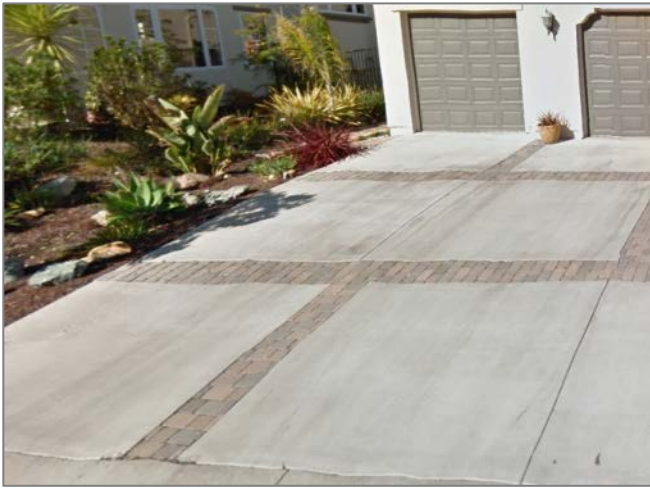
Using strips of permeable pavers to intercept runoff from large expanses of impervious surfaces disconnects these surfaces from the storm drain system.
